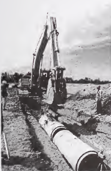
b) Laying Pipe with PipeMan
